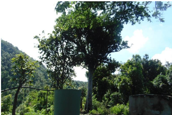
Fig 12: After the two water tanks is the flat area which is suitable of installing the solar system. However, most of the trees will be trimmed and some of them will be cut down and used as timber.
