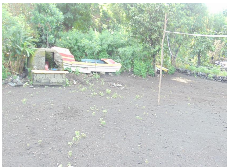
Fig 11: This installation site is on ground zero and vulnerable for sea flooding. Hence, there should be some sort of wall to prevent large waves from destroying the system.
