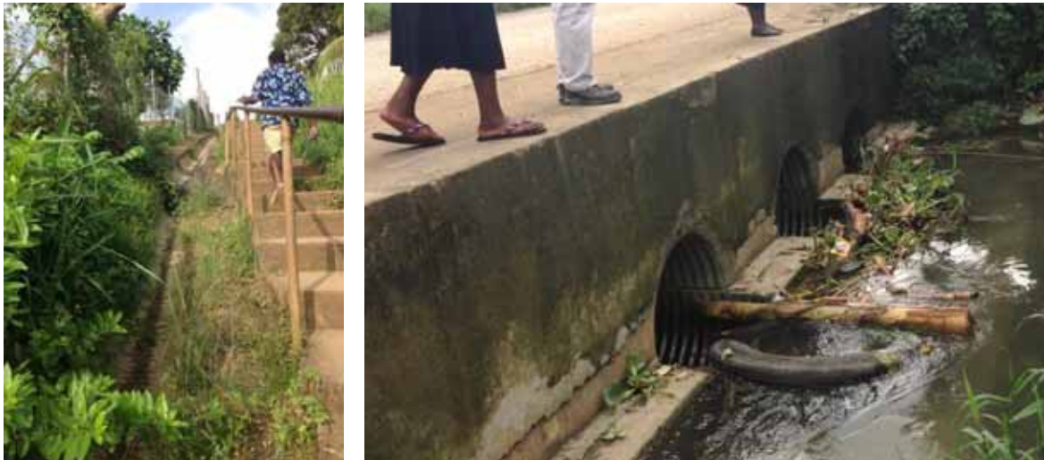
Figure 23: The 'Main Drain' below the Australian High Commission (left) and debris blocking the Tagabe River Bridge in Blacksands (right)
