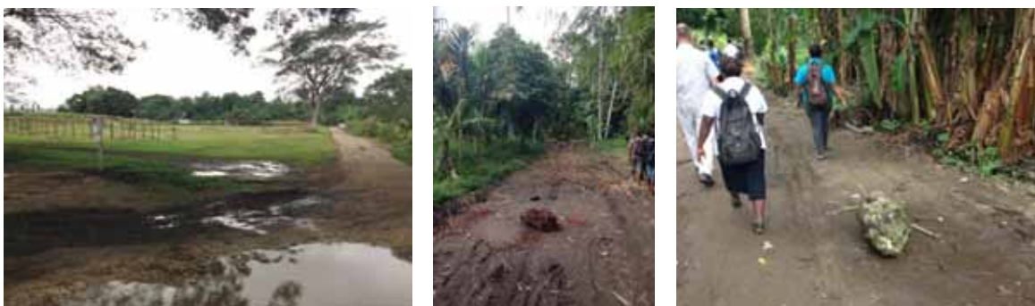
Figure 22: Unsealed road surfaces along the main road through the Blacksands informal settlement area
