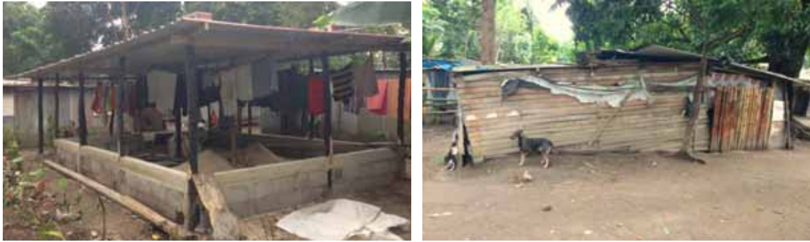
Figure 20: Incomplete concrete brick building (left) and a permanent housing structure (right) in Blacksands
