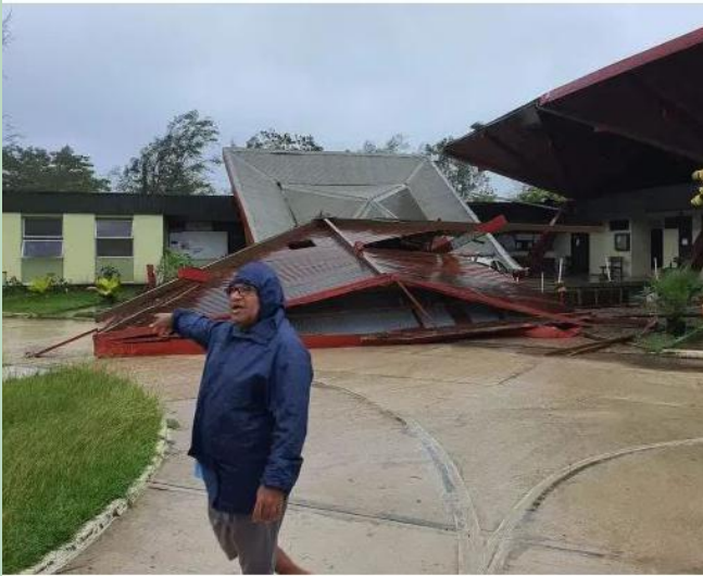
Tropical Cyclone Harold, Luganville Town, Municipal building destroyed
