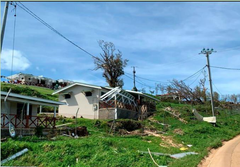
Cyclone Harold, a house damage at the VMF Barack in Santo Island Credit: AP copyright: world Vision
