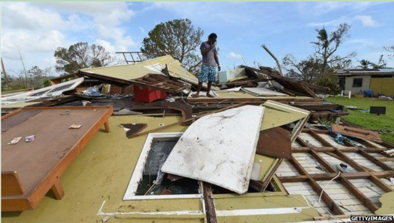
Tropical Cyclone Harold - a house fallen down and damaged. Credit: UNICEF
