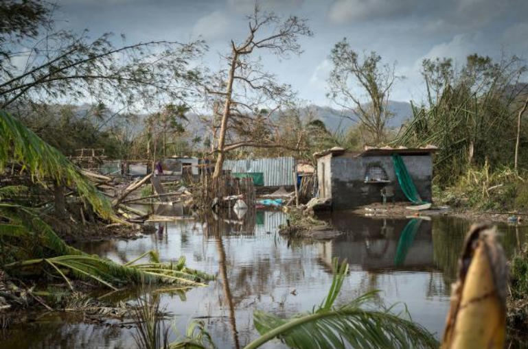
Tropical Cyclone Pam, residence suffered damaged and destruction in Efate Island: Photograph: copyright 2015 New Zealand Defense Force
