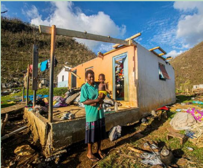
Tropical Cyclone Harold - roof of the house being blown away. Credit: UNICEF
