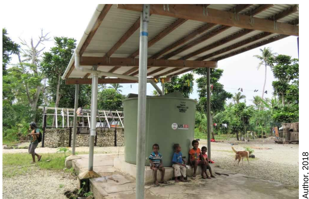
Figure 2.2 Improved tank and rainwater catchment system in Worasiviu, Pele island, Vanuatu
