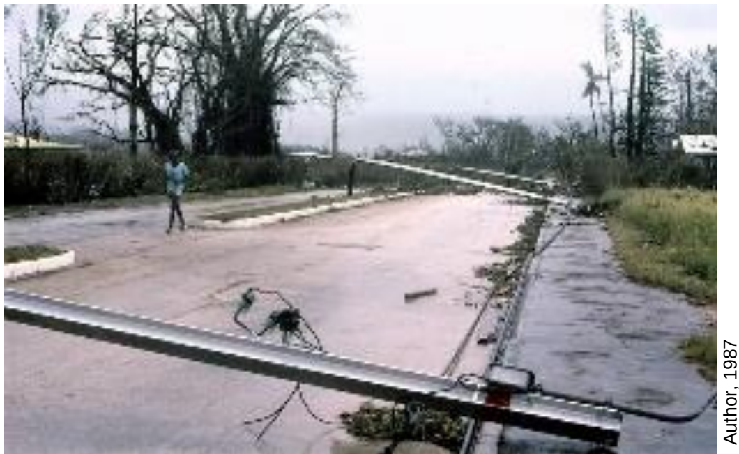
Figure 1.5 Cyclone Uma, February 1987: in Port Vila, violent winds have bent these reinforced steel utility poles down to the ground
