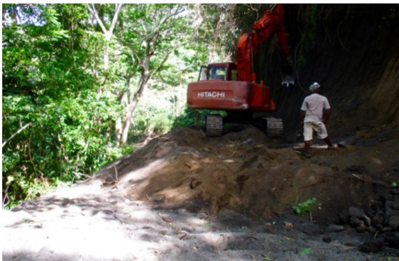
Road Repair on Pollan Hill, West Epi.
