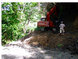
ROAD REPAIR ON EPI
