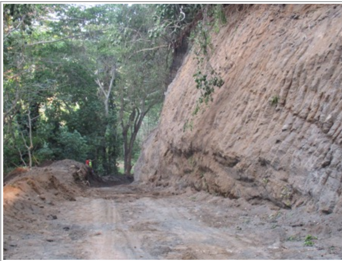
Road repair on Pollen Hill, Epi.
