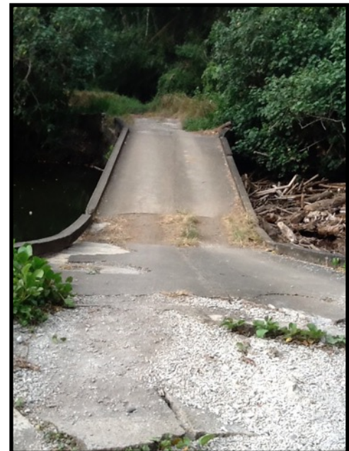
(Collapsed bridge near Yervali School)
