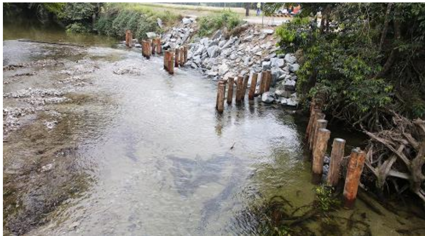
Figure 14: Example timber piles in Australia – Top: South Pine River, QLD, Bottom: Mossman, QLD
