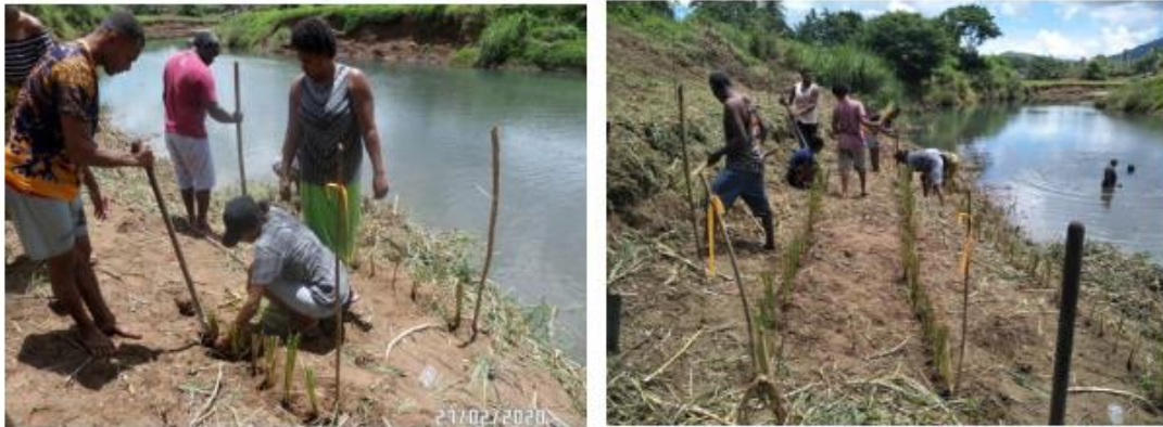
Figure 25: Preparation of furrow and planting for bank slope stabilization (Vunimoli village Labasa, Fiji)
