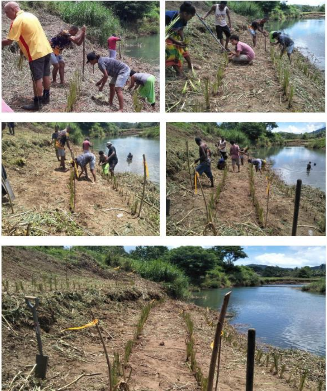
Figure 28: Vetiver propagation at a vulberbale riverbank
