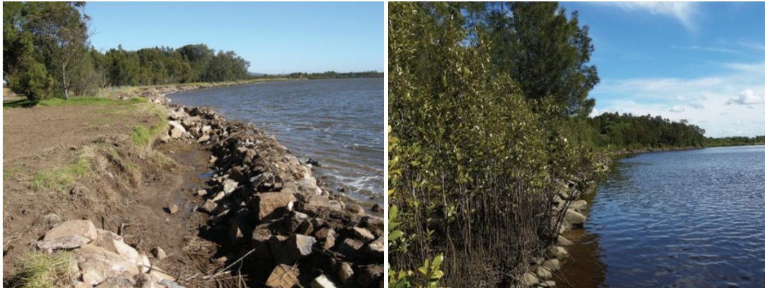
Figure 16: Typical rock fillet after construction and following mangrove establishment ((Jenkins & Russell, 2017))
