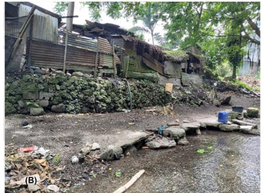
Informal housing with a greywater soak pipe discharging into the Tagabe River. Photo credit Ediza Negwele.
